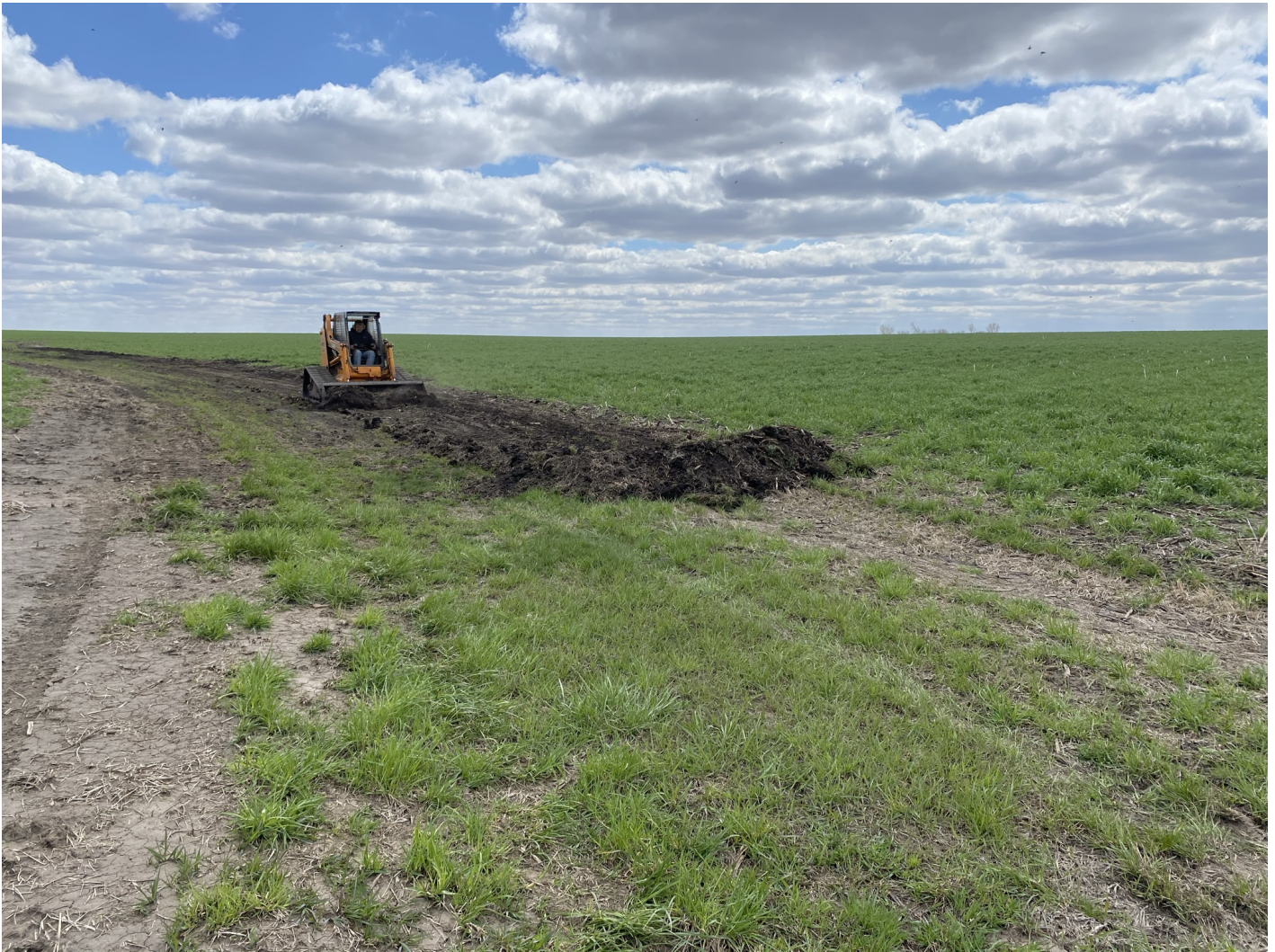
Photo: Operator is reshaping a waterway on a farm with a winter-hardy cereal rye cover crop growing. The farmer will take the excess dirt collected and fan it out into the farm field.
