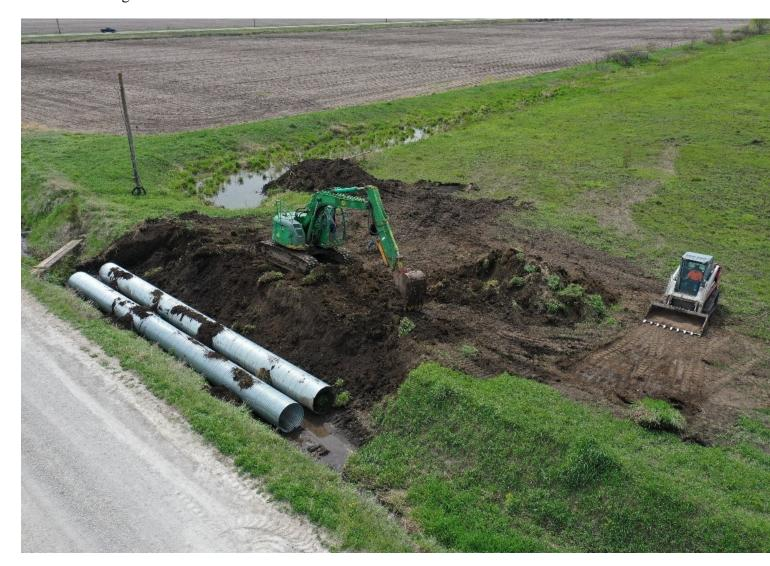
**Above:** A forty-foot field drive being installed on a Peoples Company managed farm to increase field access and safety for the operator.
