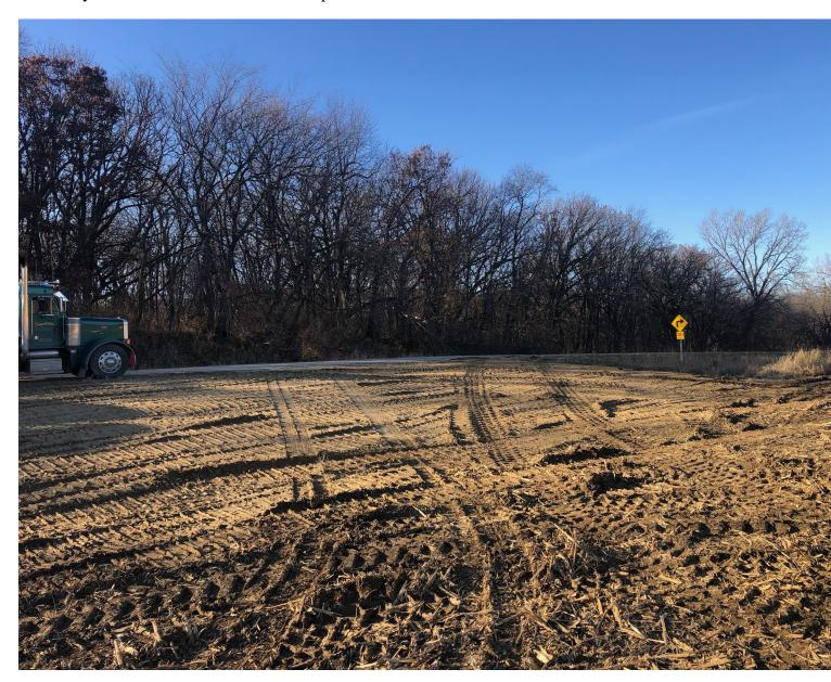
**Above:** This image was taken on a managed farm in Guthrie County, IA. The previous field driveway was 20-feet wide, on a sharp curve along a paved road. To increase safety, a new 60-foot field drive was installed to allow the farm operator easier and quicker access to the field, posing less of a threat to commuters.
